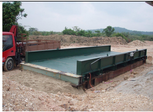
Installing Weigh Bridge
